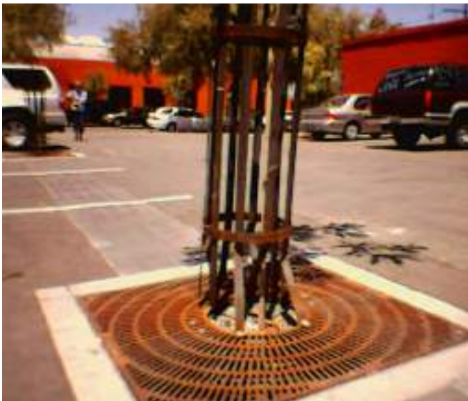
Fig 50: Palo Alto was the first western city to use the Cornell University patented method planting mix (390 Lytton—not shown) and in the above photo, structural soil 24" deep provided room for the roots of this Chinese pistache—below the parking lot surface—at another downtown location.
