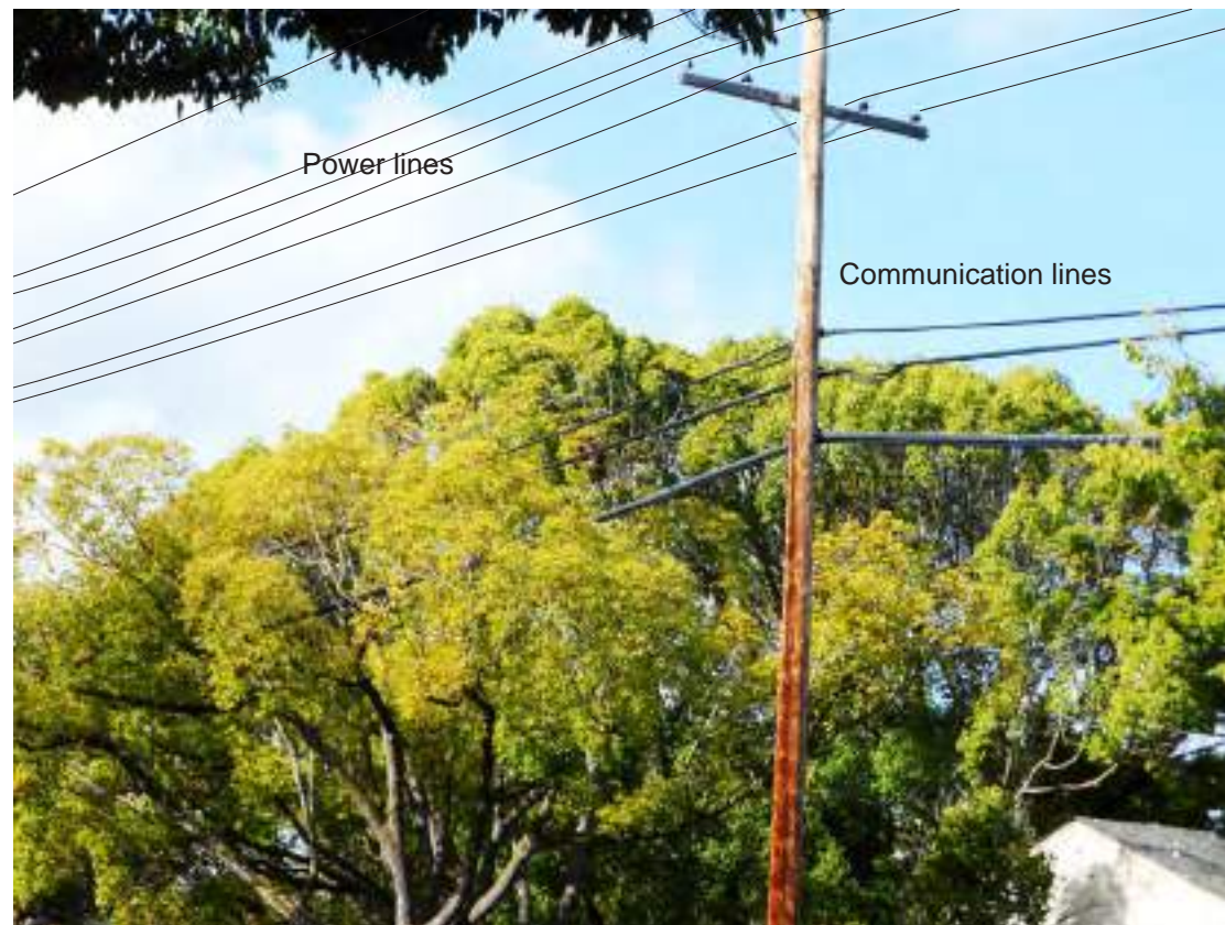
Fig. 53: Communication wires may run through canopy. However, power lines have strict clearance requirements established by the California Public Utility Commission.
