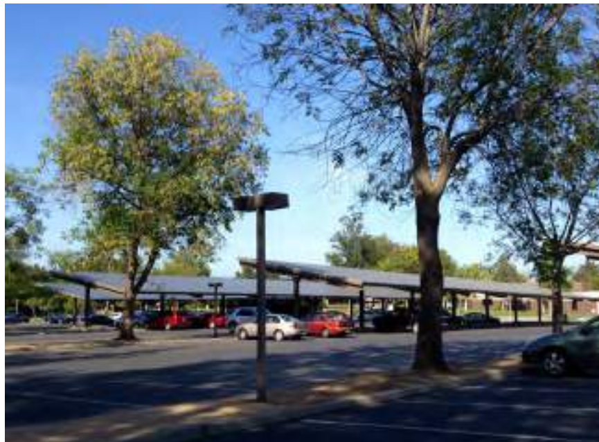
Fig 43b: This West Valley College parking lot provides a local example of a partial conversion from shade trees to solar panels.
